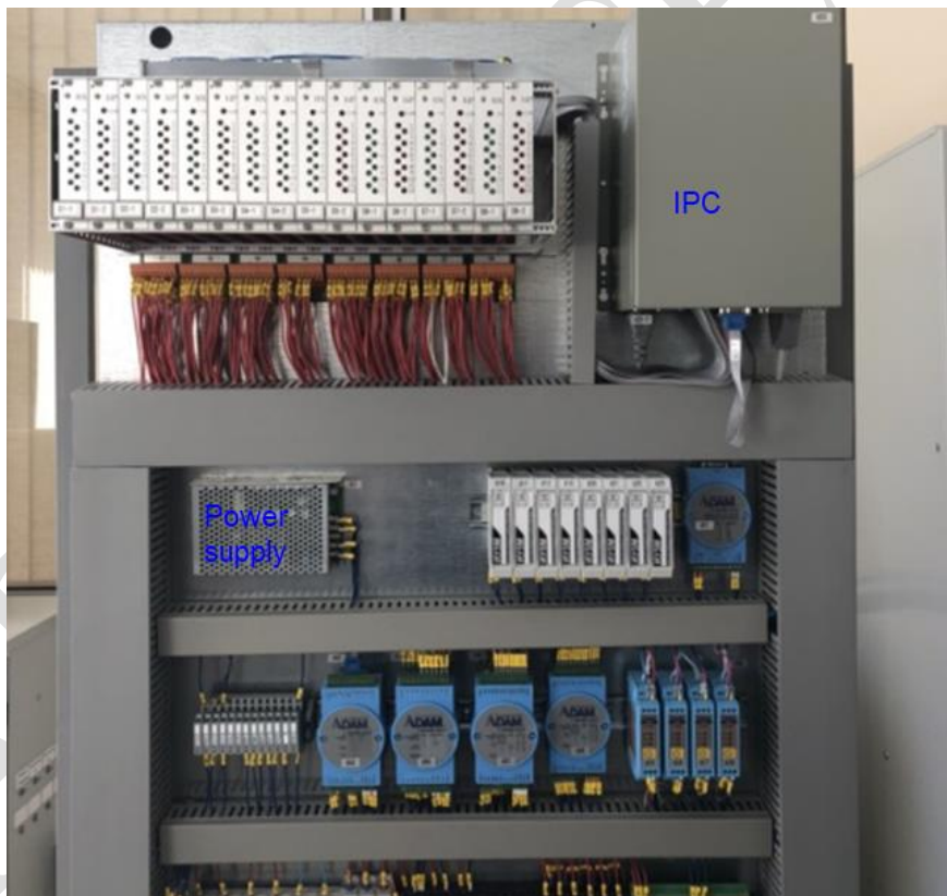
Figure 2 A good way to install and use ADAM module in a control cabinet
