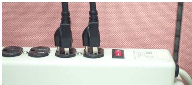
Figure 3.12 Power cord plugs should have same orientation in socket/ 插座上电源线方向相同 / 插座上的電源線方向應相同
